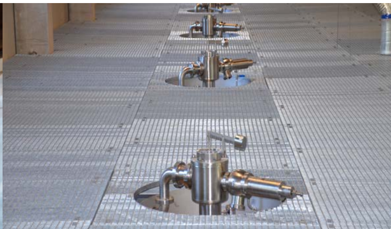
↖ Safety valve on a bioreactor
